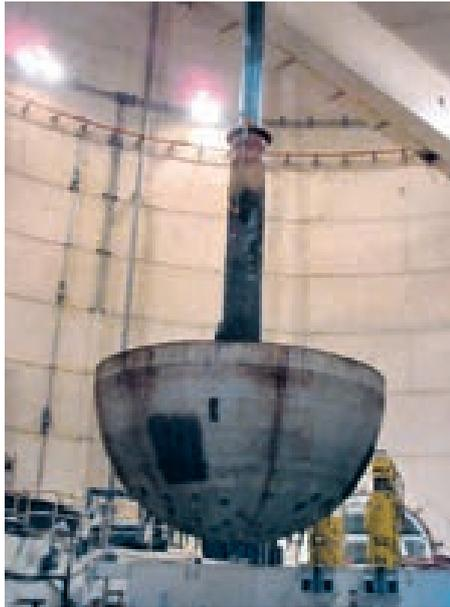
Reactor floor on a lifting rod
