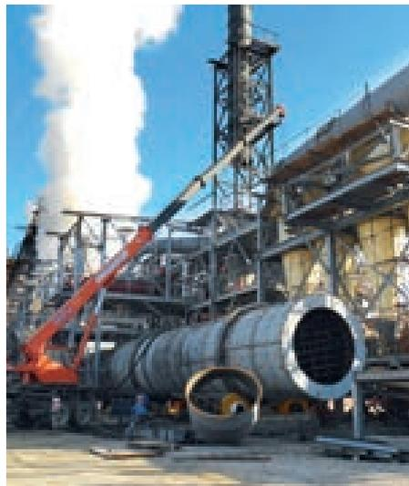
The drying drum is brought into position in front of the already installed combustion chamber
